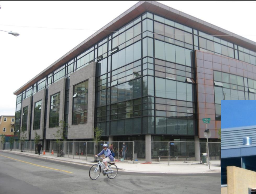
Dalhousie New Academic Building
